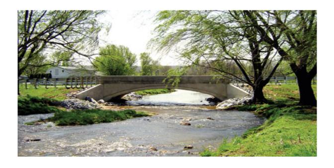
The best type of stream crossing structure that allows for unobstructed fish passage is a bridge. However, it is very expensive to justify this type of installation for streams having a drainage area of less than 20 km<sup>2</sup>.
