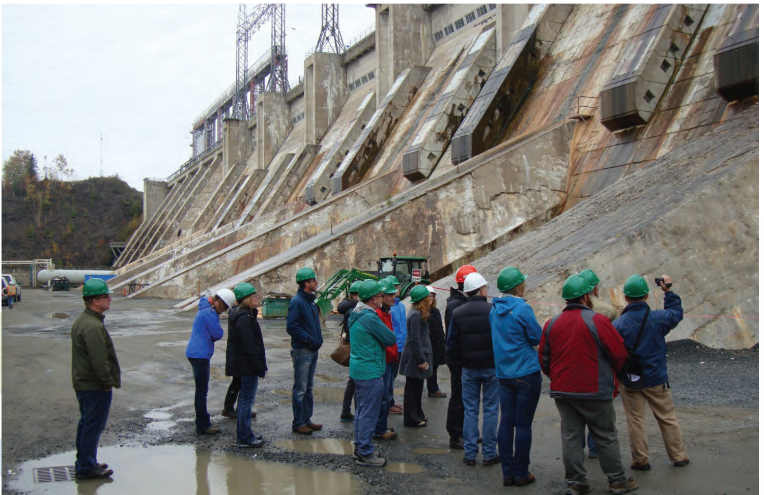
NB Power's Mactaquac Dam
