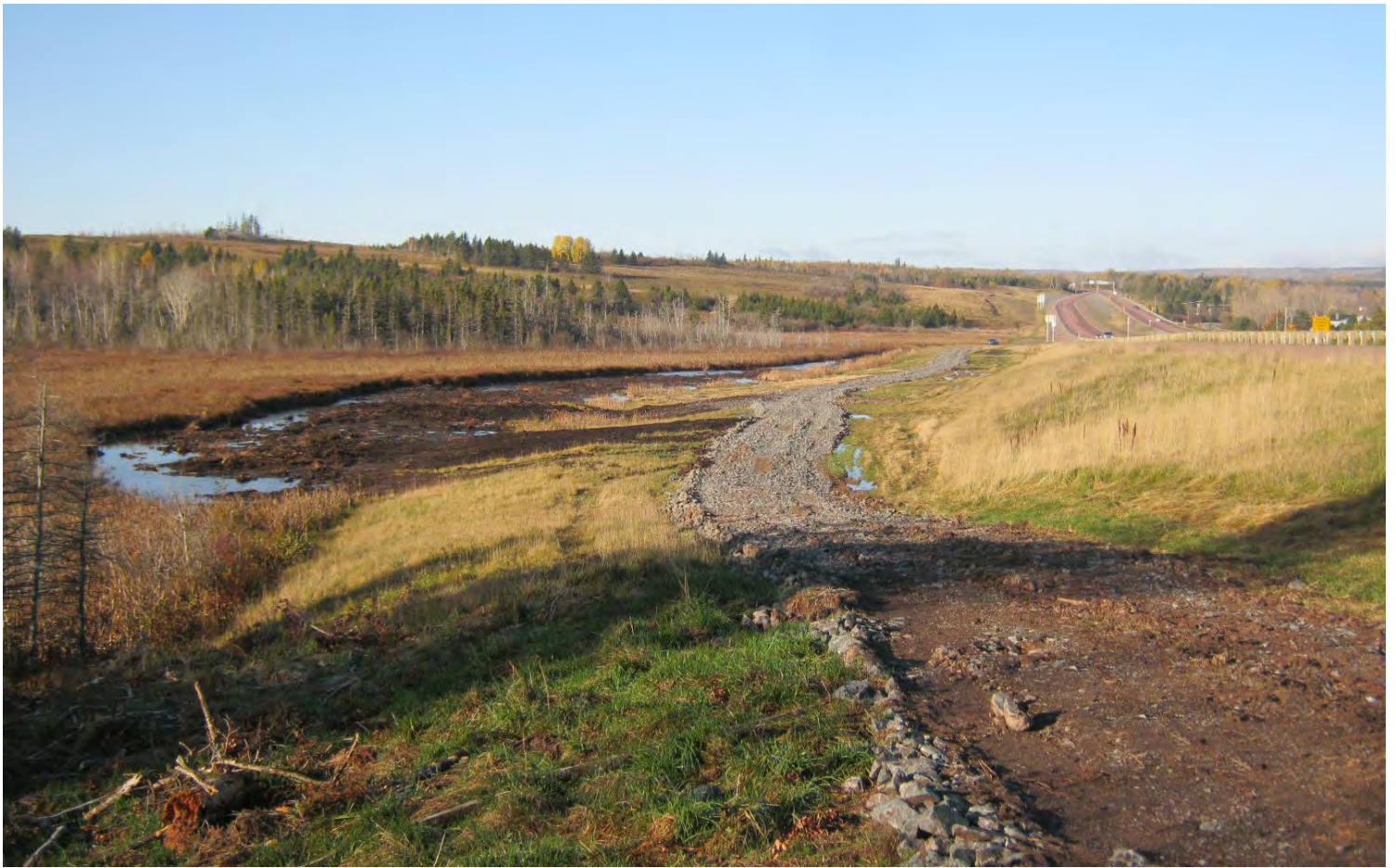
Figure 5 Site overview at completion (October 2013). Berm slopes remain vegetated and largely undisturbed, temporary gravel road remains in place. Irregular surface of recovered portion of wetland will facilitate vegetation recovery and adaptability of community to changing conditions.
