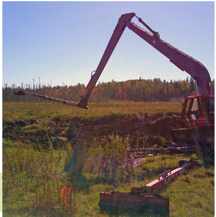
Figure 3 - Linkbelt 3400 LII Long Reach excavator with extension
